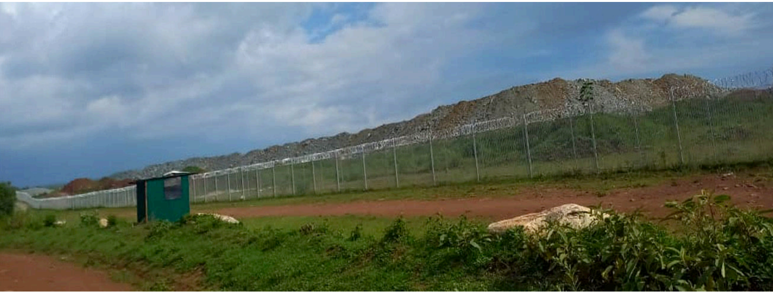
Photo: New fence and guard posts around cleared land and new pit construction. November 2023. MiningWatch Canada
