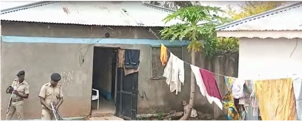
Photo: Police overseeing the bulldozing of houses in Komarera Village. December 2022. (Still from video with MiningWatch)
